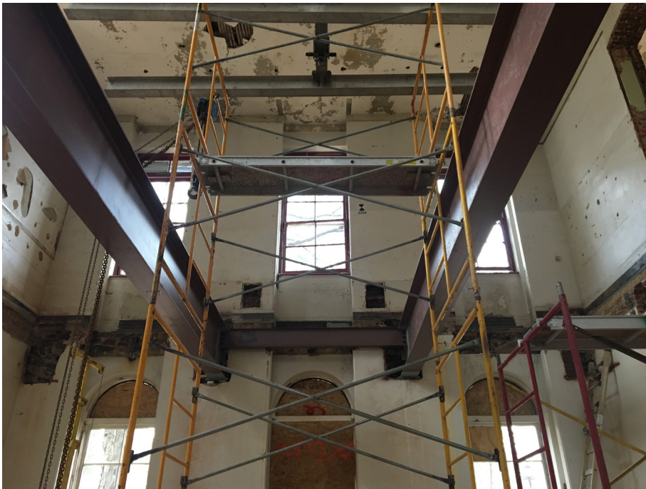
Existing floor framing and support columns were removed, with new floor framing (below) allowing for the creation of an open classroom space.
