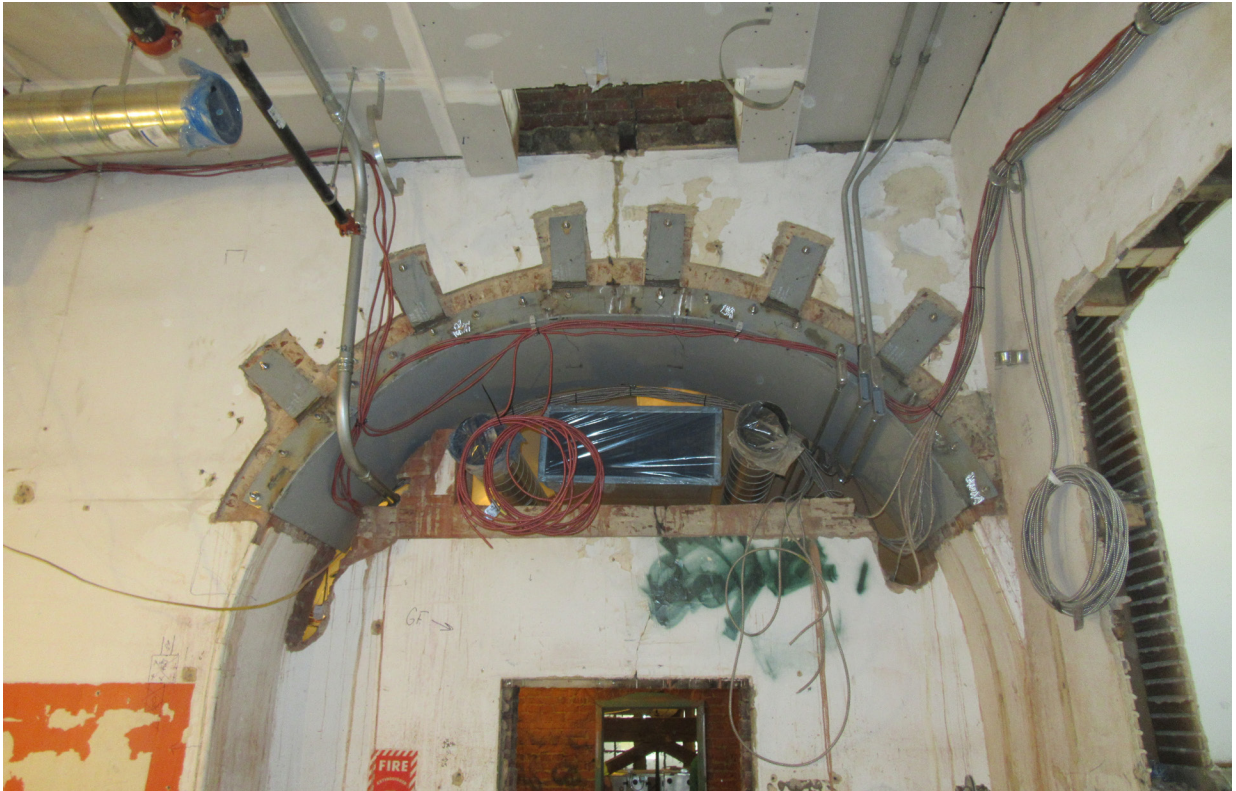
Opening created in 32"-thick masonry wall with new lintel.
